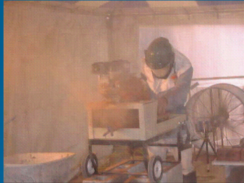
No dust control
